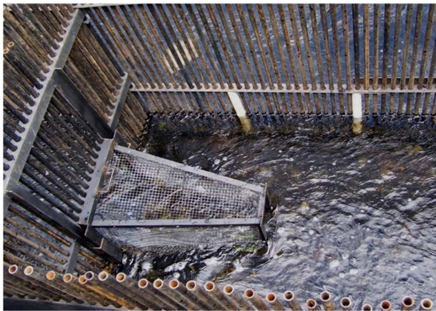
Figure 7. Top view of the fyke inside the collection box.
