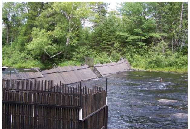
Figure 17. View of support cables connected to the weir panels and upstream portion of the collection box.
