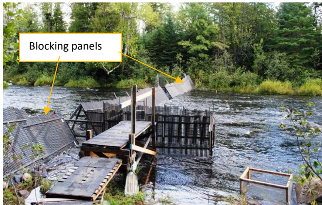
Figure 5. View of blocking panels spanning the stream.
