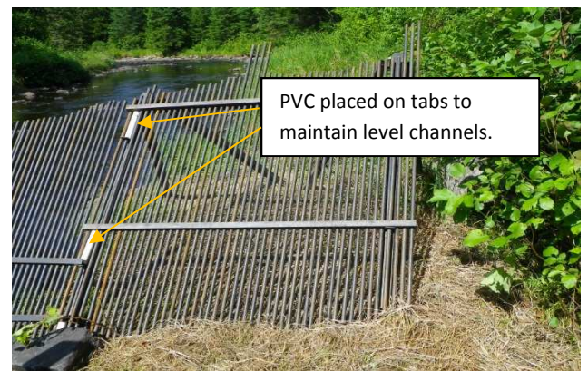
Figure 15. Use of PVC sections, resting on tab of front tripod leg to maintain level channels in the blocking panel when moving up the streambank.
