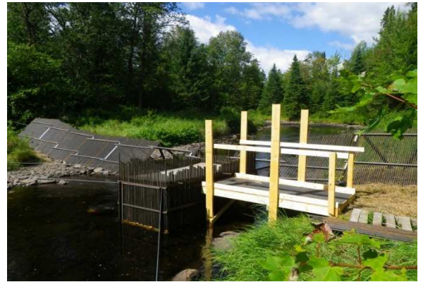
Figure 18. Walkway/work platform extending from the streambank to the collection box.
