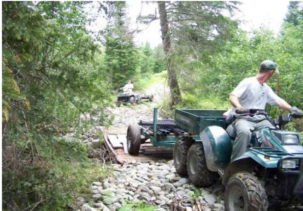
Figure 13. Transporting material to the weir site using ATV's and trailers.
